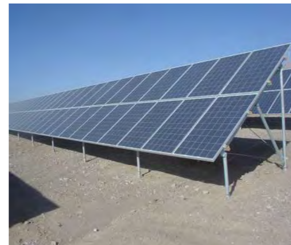
Project Location: Africa Capacity: 1.6MWp Completion Year: 2015 Type: Ground Mounted
