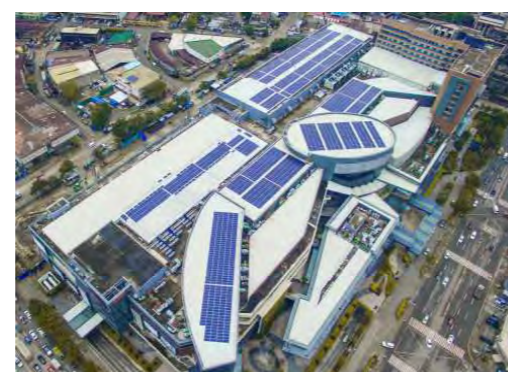
Project Location: Cebu, Philippines Capacity: 2.5MWp Completion Year: 2017 Type: Metal roof Mounted
